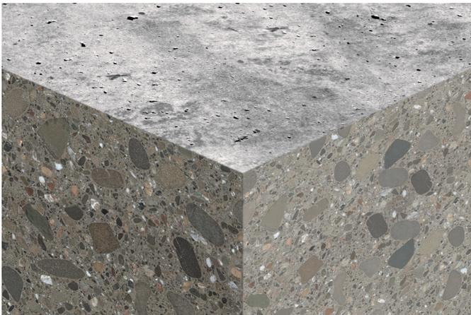
LI/LIP concrete in general is a type of concrete with optimised resistance against penetration by water polluting substances. LIP concrete is a liquid impermeable concrete after penetration testing. LI/LIP concrete is designed so as to be considered liquid impermeable.
