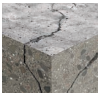
Cracked concrete
