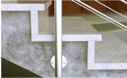
Handrail anchorages
