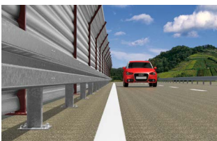
Sound insulation walls
