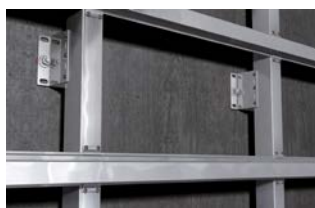
Facade substructure
