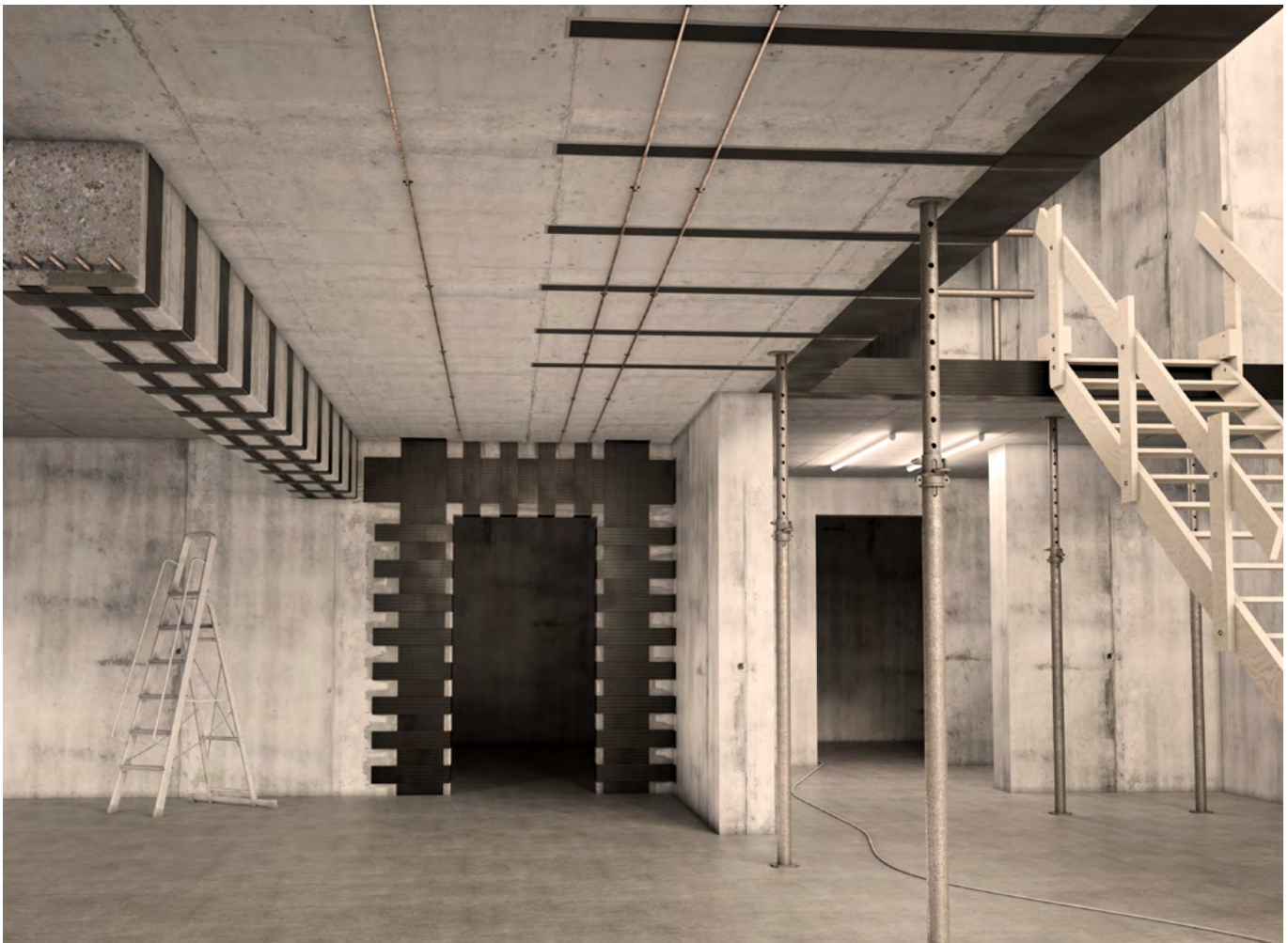
Fig. 1 – Building with flexural and shear strengthening
