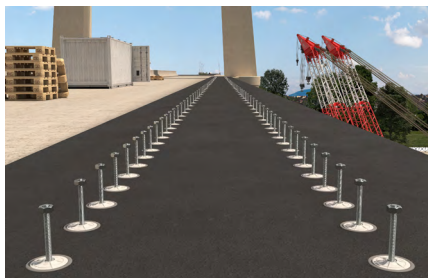
Bridge cap anchor with nut
