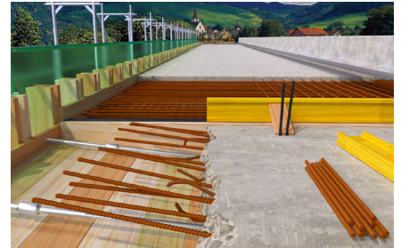
Rebar connections
