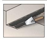
A scratch coat of FRS-CS should be applied to the concrete surface and the CFRP Laminate applied wet-in-wet.
