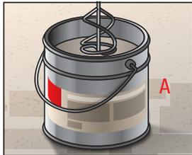
The FRS-CF 2-component epoxy saturating resin must be prepared by following the processing steps in accordance with the Technical Data Sheet (TDS) of FRS-CF. Note the required mixing ratio, pot life, storage temperature and the proper mixing procedure.
