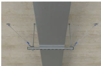
Lateral bracing of ventilation ducts
