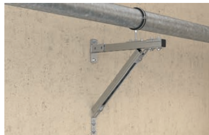
Upright pipe on cantilever arm
