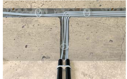
Cable fixing in wall slots < 55 mm
