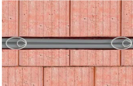
Cable fixing in wall slots > 30 mm
