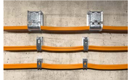
Cable fixing to the wall
