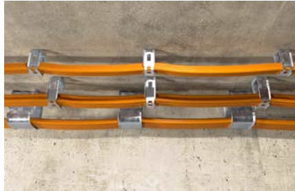
Cable fixing to the ceiling
