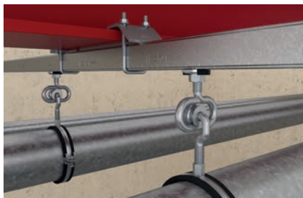
Channel fixing to steel beam
