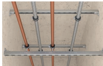
Pipe fixing in a corridor
