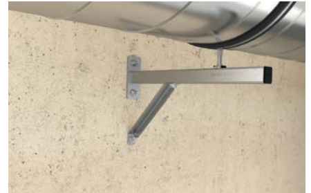
Ventilating pipe fixing at the wall
