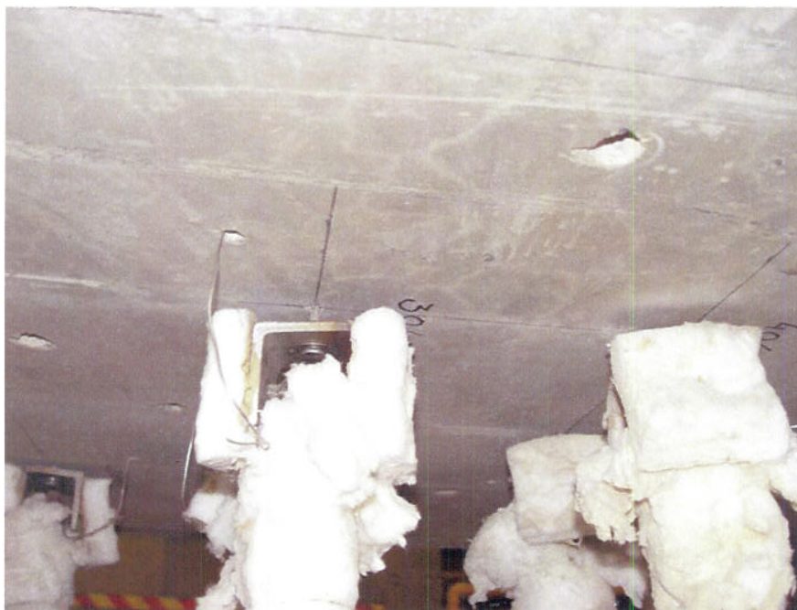
Photo 2 : detailed view of one of the anchors
